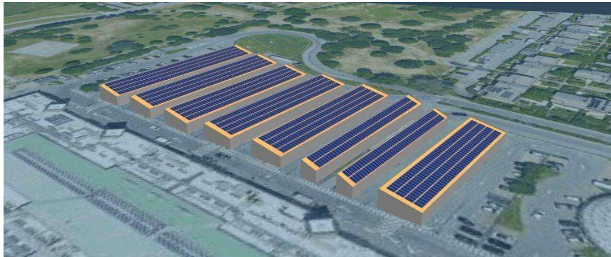
Collective Self-Consumption Project: PV system on parking area shelters. Via Larga Shopping Center, Bologna
